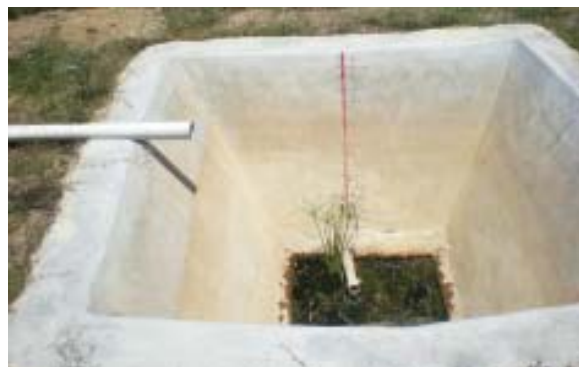
Plate 5. Outlet for gravity fed irrigation system inside the reinforced plastered lined tank
