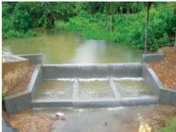
Plate 4. Construction of check dam and installation of observation well
