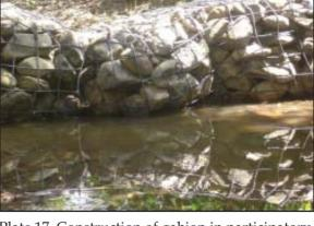
Plate 17. Construction of gabion in participatory mode through Water Users Association
