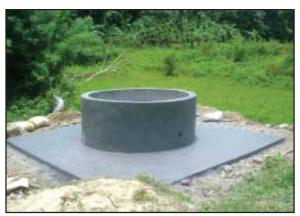
Plate 16. Construction of ring well for irrigation and drinking in participatory mode through Water Users Association
