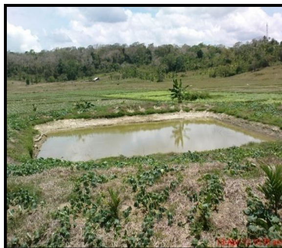
Fig 31. Water harvesting structure Tank cum well system
